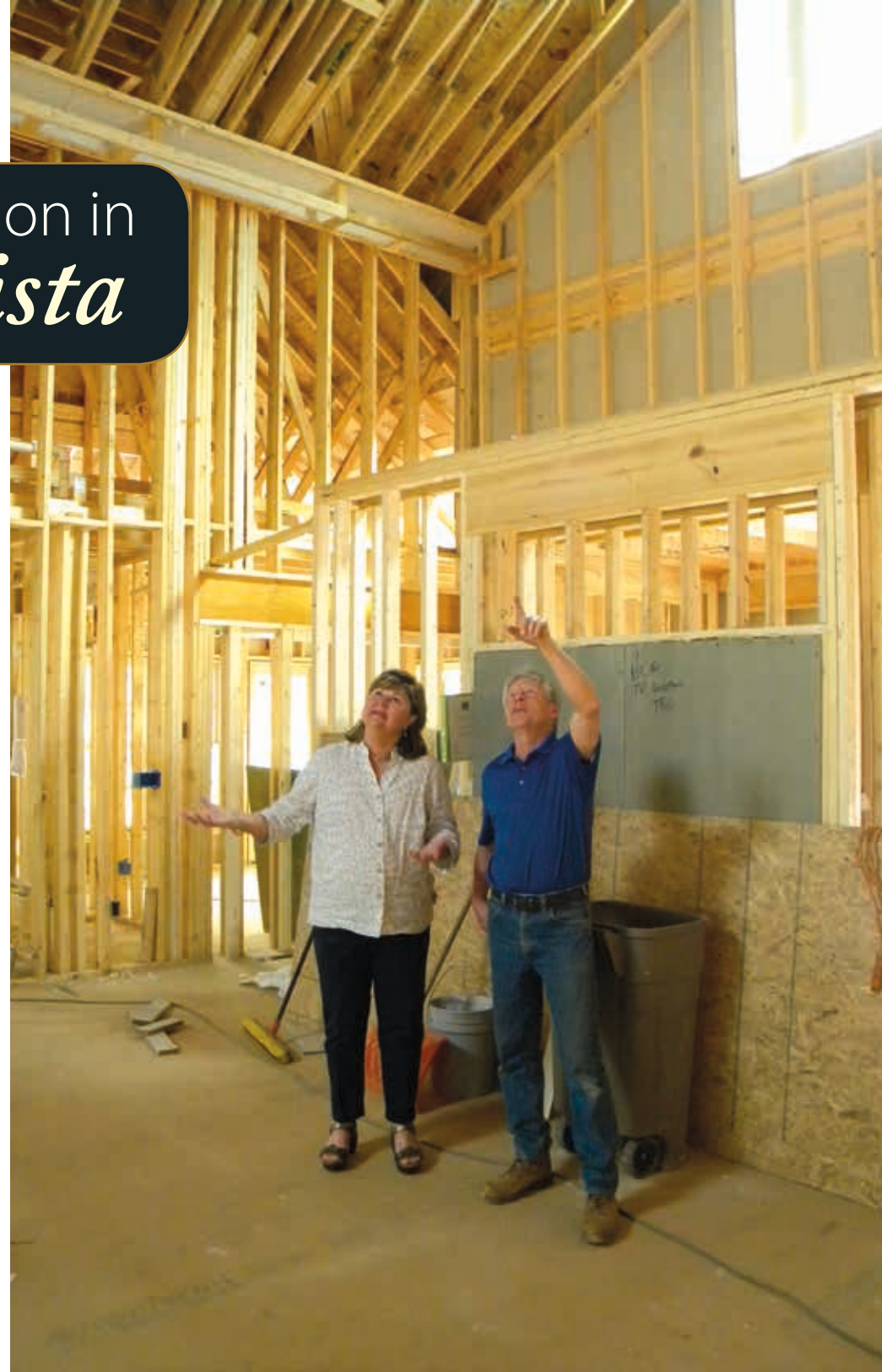
June and Don discuss the interior vaulted ceiling.
